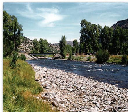
1998. Lake Fork near Cross Section 2 following reconfiguration. The cobble bar forming the left bank was constructed of material dredged from the streambed to the right. The large, partly submerged boulders in the channel were quarried off site and added to the streambed during reconfiguration. Discharge is 230 ft<sup>3</sup>/s.
